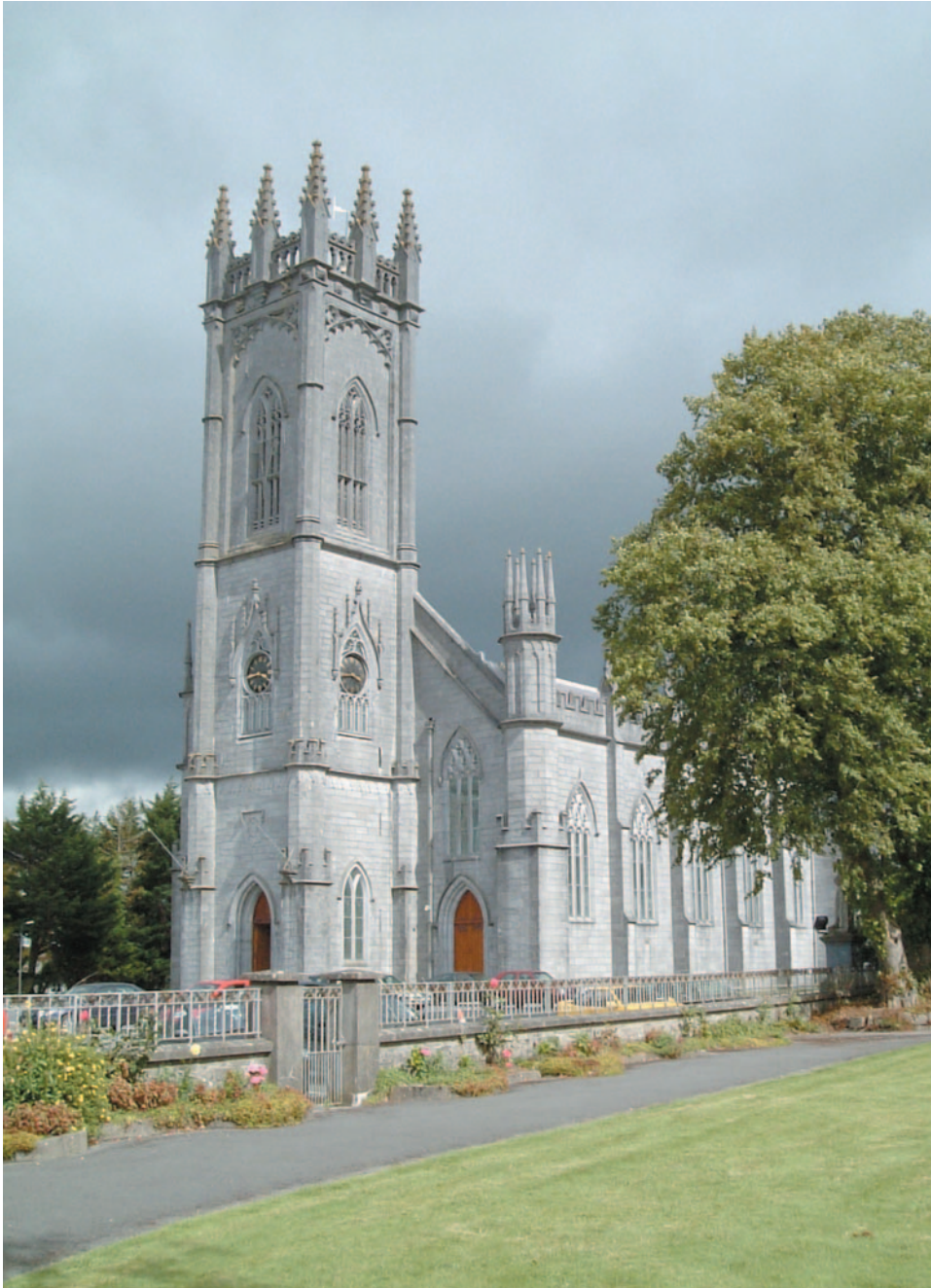
1 – Dominick and Peter Madden, Cathedral of St Jarlath, Tuam (1827-36): view of west front (photo K. Mulligan)
