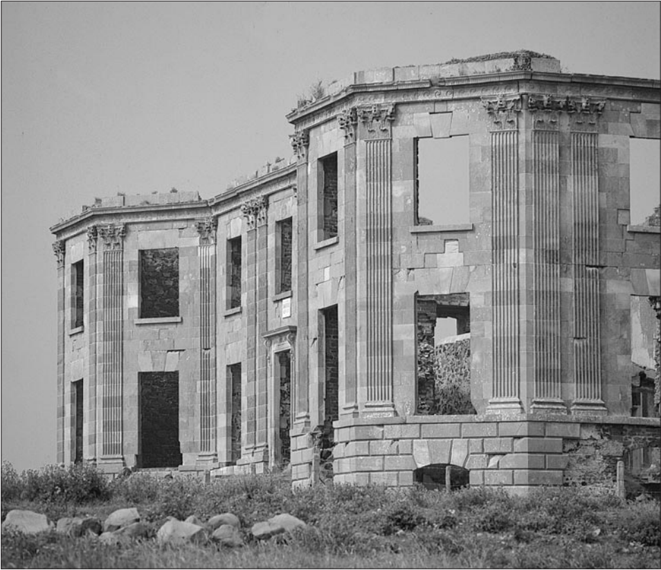
2 – View of Downhill, county Londonderry, in its ruined state (courtesy National Trust Photographic Library; photo Mike Williams)
