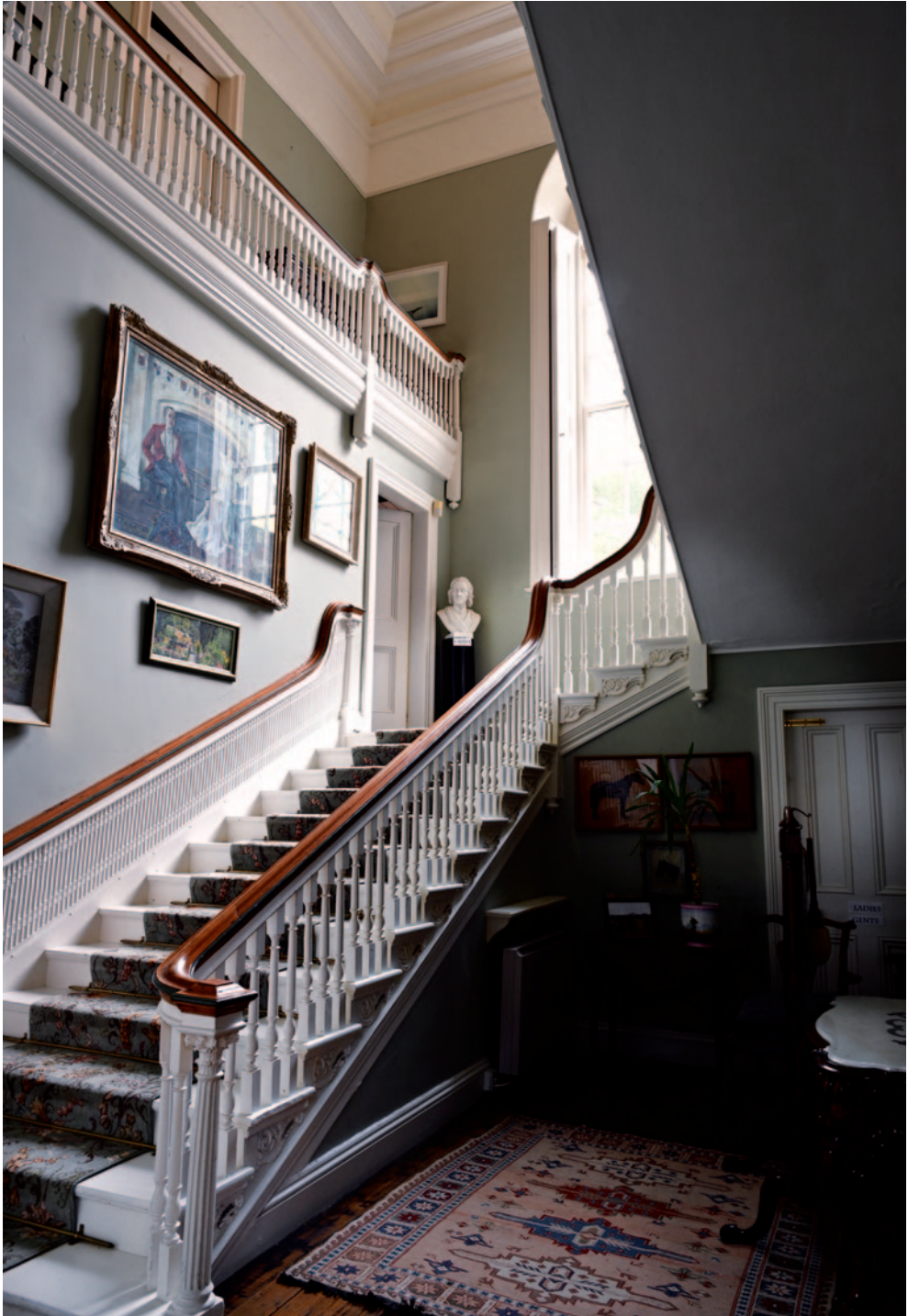
9 – Lord Ferrard's new staircase hall at Beaulieu House viewed from below, with its round-headed window, timber cornice, and Dublin-made cut-string staircase of 1722-23
