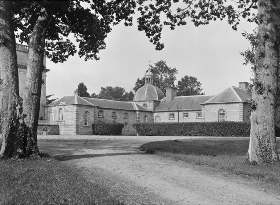
29 – Castletown, Carrick-on-Suir: use of domed pavilion and the deployment of wings in an inward-turning L-plan to partially enclose a yard (courtesy Country Life)
