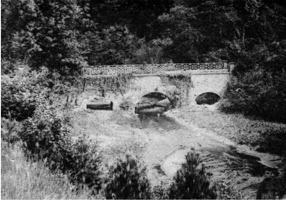
38 – Lissan Demesne, Cookstown: the bridge, c.1900 (courtesy Trustees of Lissan Estate)
