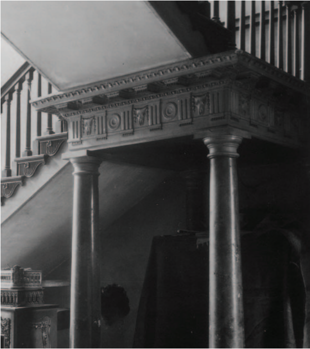
25 – Brockley Park, Stradbally: staircase with supporting columns, frieze and cornice (demolished 1944)
