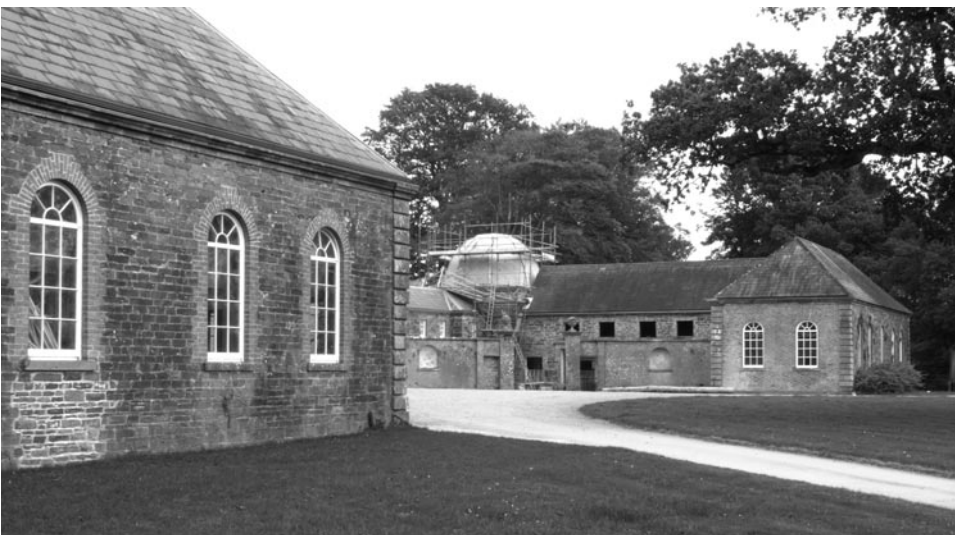
30 – Kilshannig, Rathcormac: use of domed pavilion, the deployment of wings in an inward-turning L-plan, and a curtain wall to enclose a yard (photo Dara McGrath, 2007)
