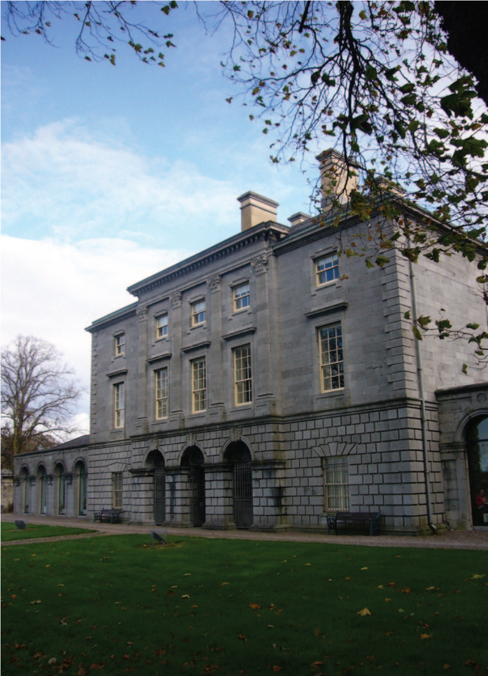
28 – Custom House Limerick (begun 1764): ‘frontispiece of fluted pilasters, arcaded wings, panelled piers, arches ornamented by a tangent circle above, concave weatherings to window cornices, and window architraves broken upwards’ (2007)
