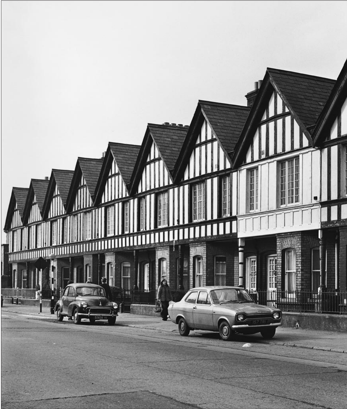
8 – Company houses from the Rialto scheme, facing South Circular Road, Dublin The architectural style adopted for this row of houses is unique amongst the Company's schemes.
