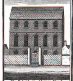
The Hospital in Stevens Street
