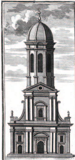
The Front of St. Warburgh Church.
