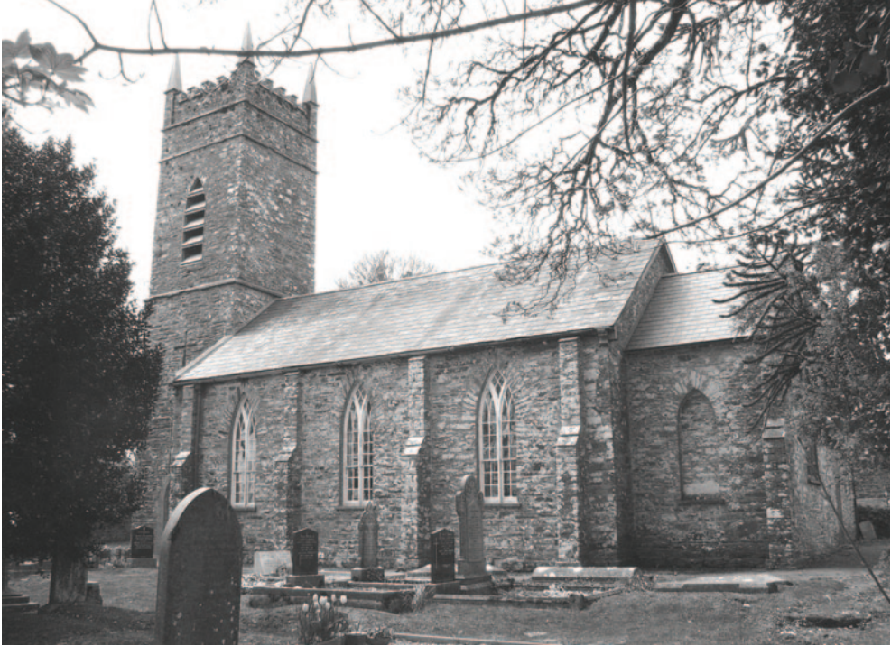
12 – Church of Ireland church, Castleventry, county Cork – view from the south-east
