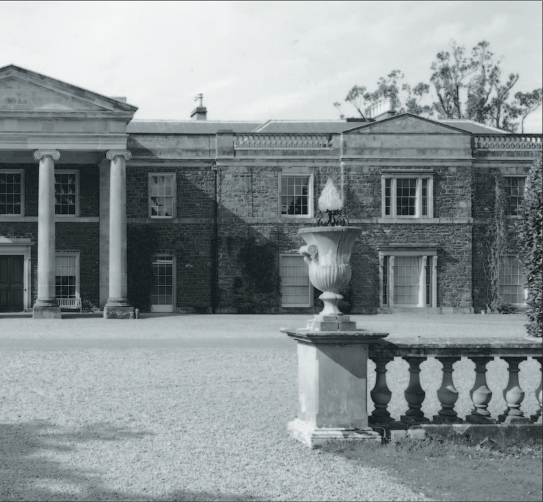
2 – North front of Mount Stewart, county Down (courtesy Anthony C.W. Merrick)
