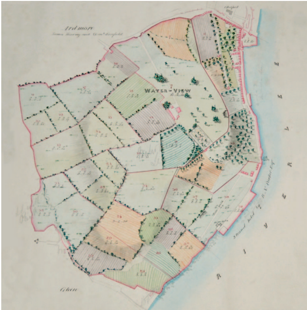
4 – Sherrard & Brassington, 'Survey of Monkstown, Cork, the joint estate of Thomas, Earl of Longford and John, Lord Viscount de Vesci', 1805, showing the townland of Maulbaun, Waterview House and the village of Passage (Pakenham Papers)
