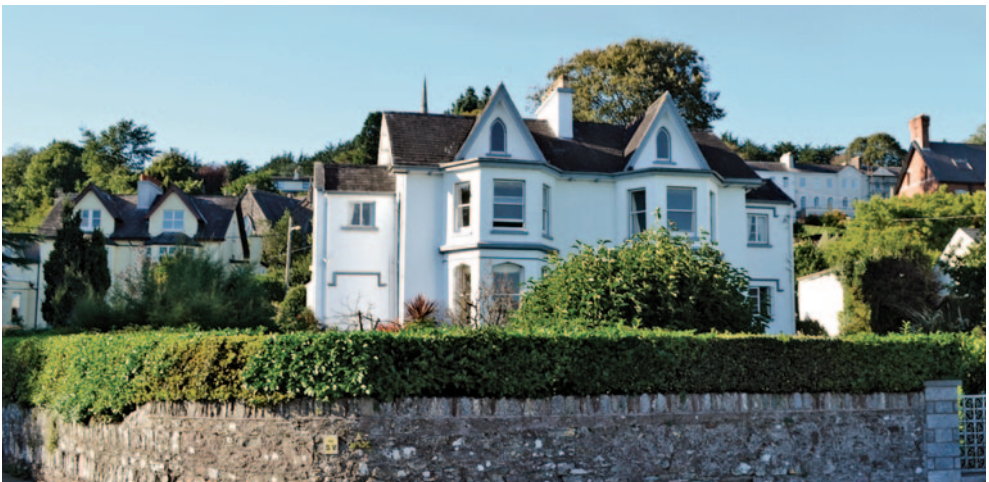
13 – Alta Terrace, Monkstown, east elevation (photographed October 2017)
