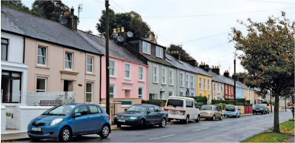
9 – Nos 1-16 Maulbaun Terrace, Glenbrook (photographed October 2017)
