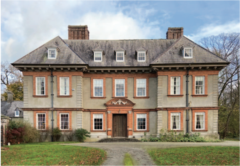
2 – Carolean classicism: the entrance front of Beaulieu House, Co Louth, begun in 1680/81, attributed to ‘John Curle of Bewly mason’ (photos by Dermott & Wendy Dunbar, unless otherwise stated)
