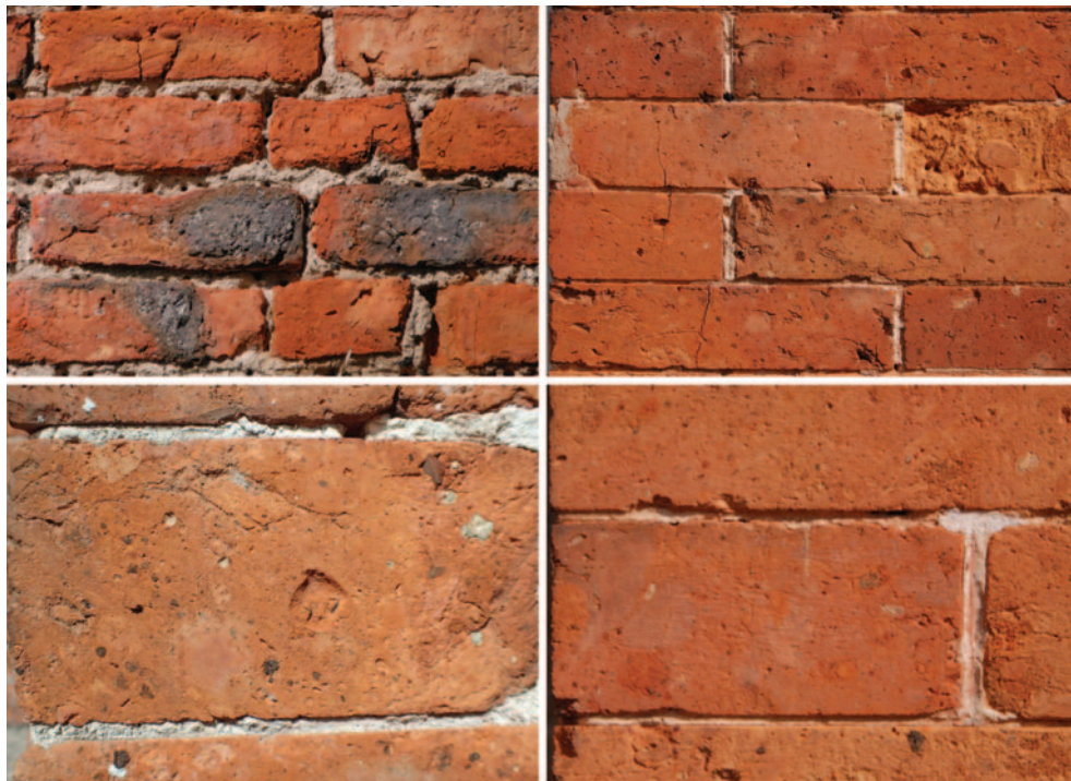
10 – Beaulieu House, uncut and cut-and-gauged bricks (photos by Jason Bolton)
