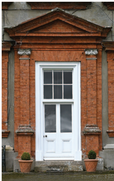
10 – Beaulieu House, uncut and cut-and-gauged bricks (photos by Jason Bolton)
