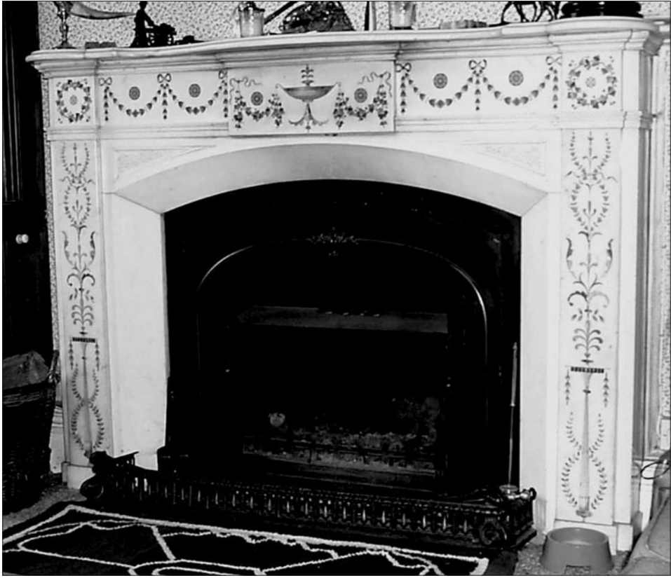
11 – Chimney piece reconstructed by Daniel Robertson (c.1840s), with scagliola inlay work attributed to Bartoli
