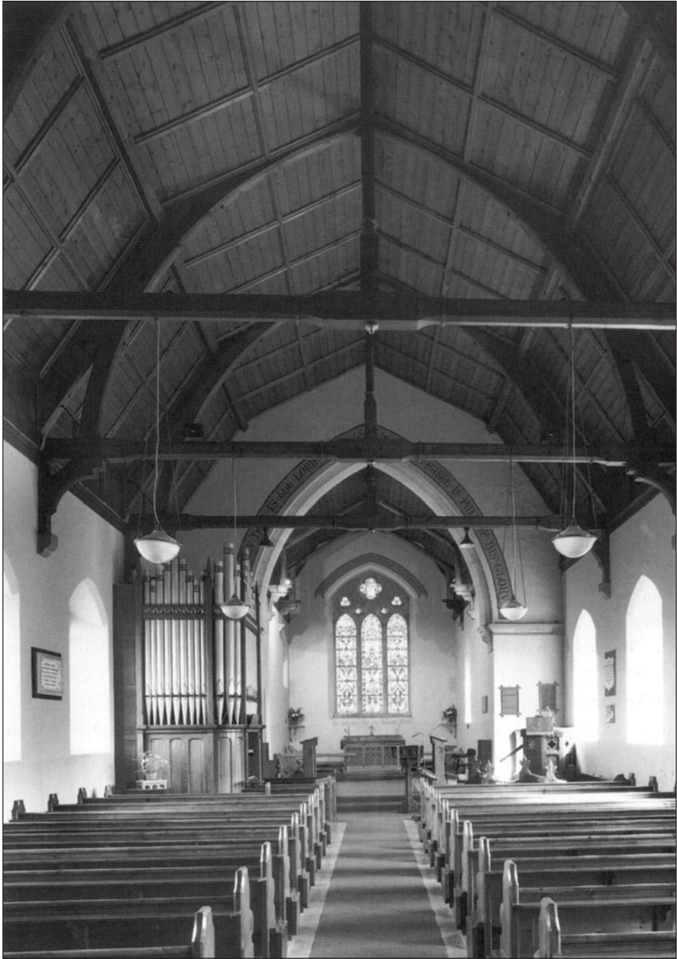
Holmpatrick church, Skerries, Co Dublin (opposite) 13 – plan (above) 14 – view of interior (overleaf) 15 – spire
