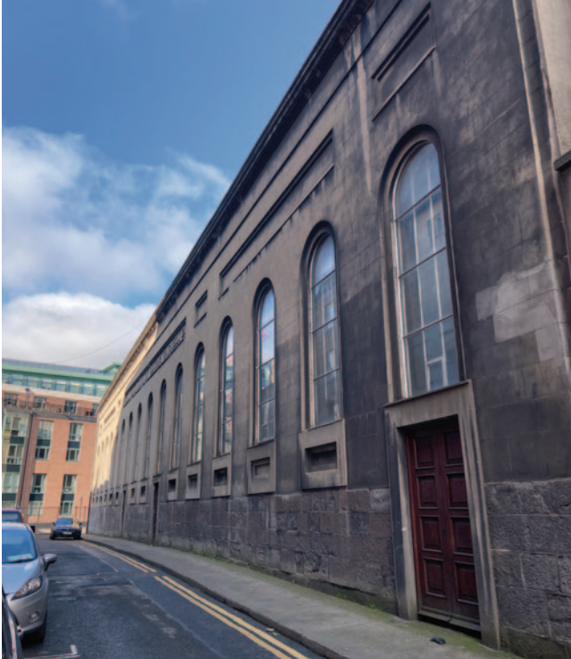
4 – Current exterior of the southern façade of the Whitefriar Street church, taken from Aungier Street
