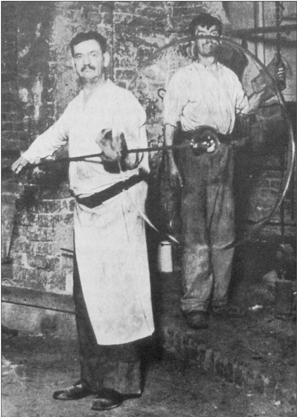
4 – A table of crown glass attached to the punty (photo from Raymond McGrath, Glass in Architecture, London 1937)
