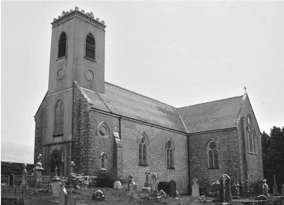
7 – St Mary's Church, Mount Bellew, county Galway: tower and nave by Dominick Madden, 1820-22
