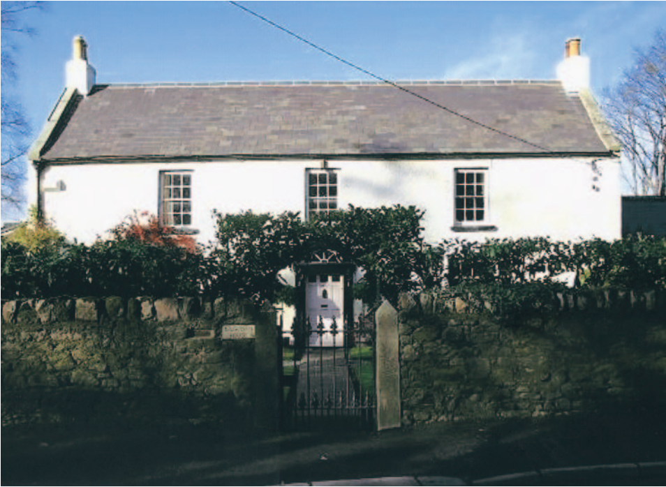
4 – Kilgobbin House, near Sandyford, county Dublin.
