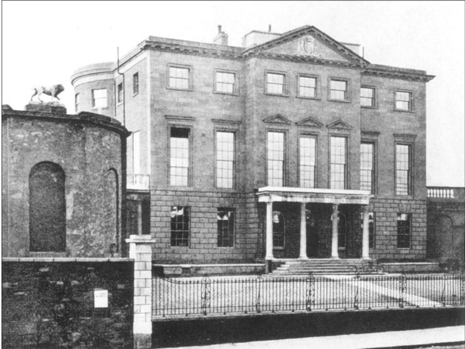
25 – Aldborough House, entrance front, c.1912
