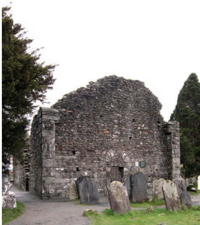
5 – Glendalough Cathedral, county Wicklow, tenth-century west façade, with antae typical of the period
