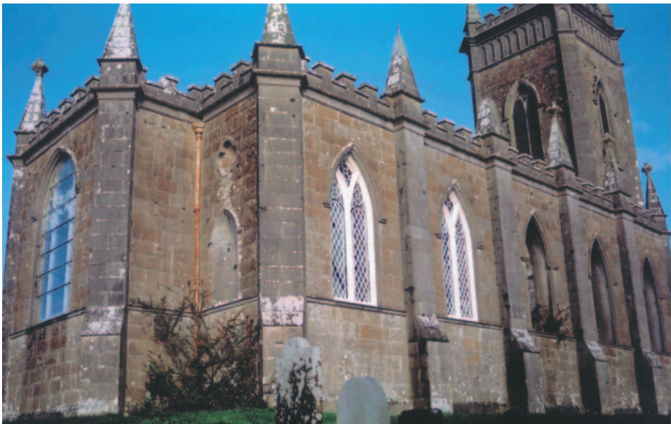
4 – Kilbixy church chancel from the south-west (photo T.S. Moore)
