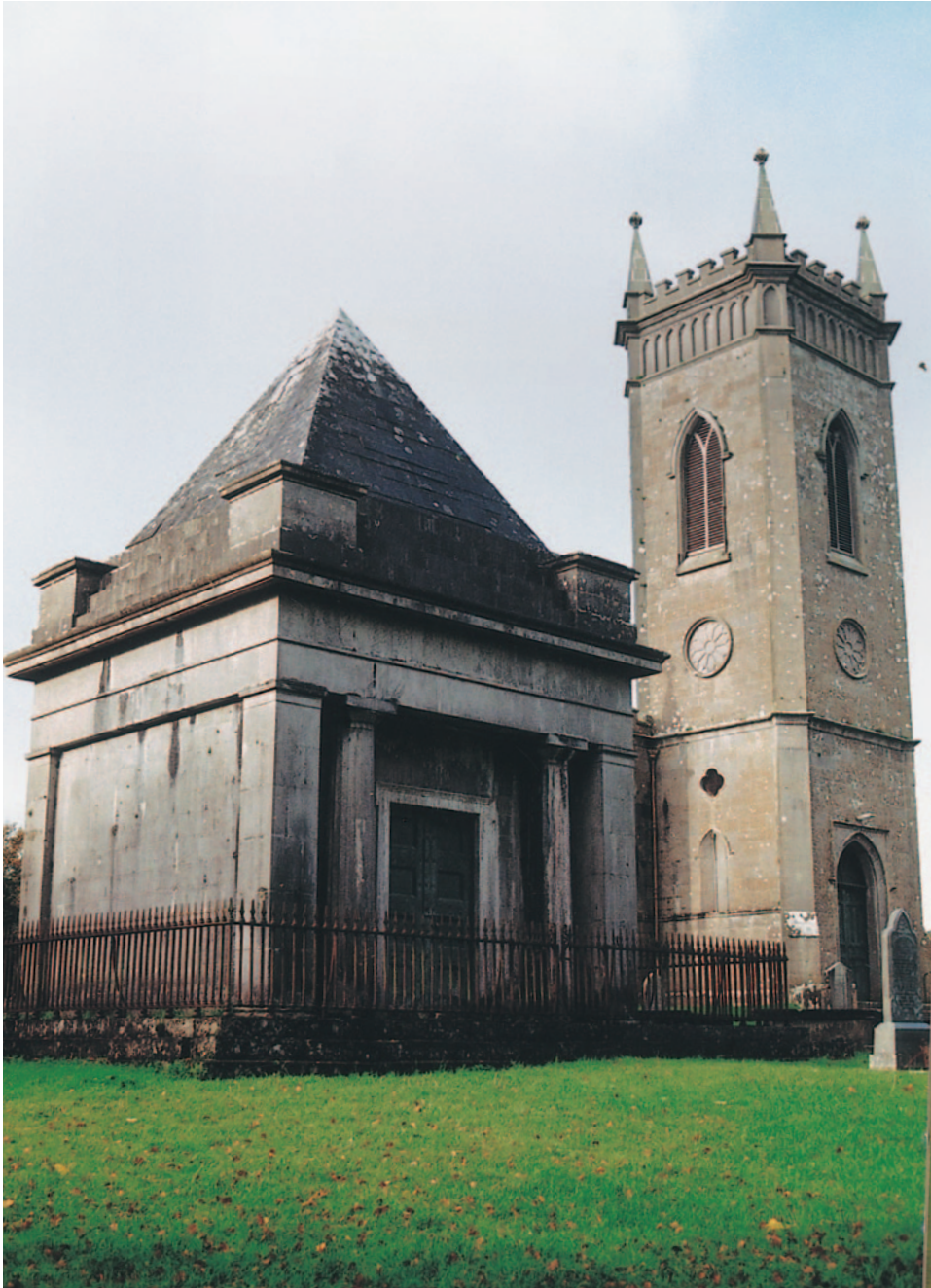
11 – Malone Mausoleum doorway flanked by footless Doric columns in antis, viewed from the east (photo T.S. Moore)
