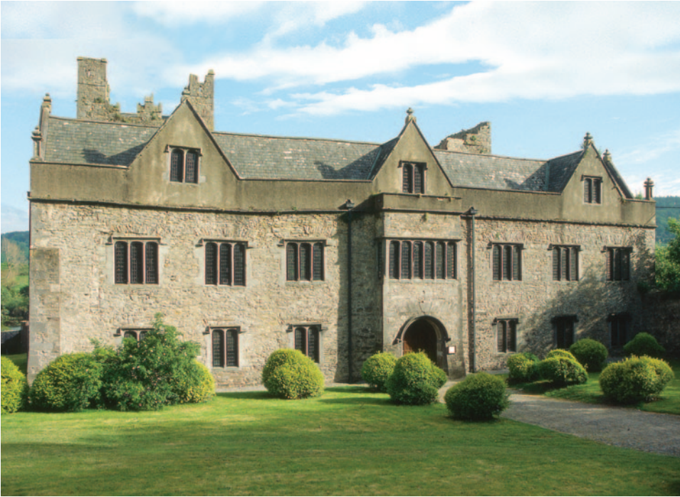
2 – Principal elevation of Ormond Castle, Carrick on Suir (courtesy Dept of the Environment, Heritage and Local Government; photo Con Brogan)
