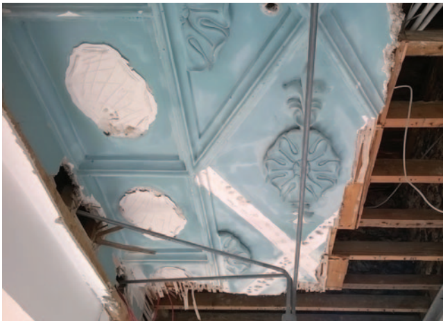
17 – Compartmented ceiling in the ballroom
