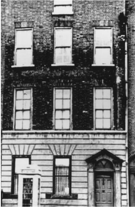
3 – Mr Stern Tighe’s house on Usher’s Quay It is now demolished. The downpipe on the right was made from marble, eight inches square and in lengths of three feet (courtesy Irish Architectural Archive)
