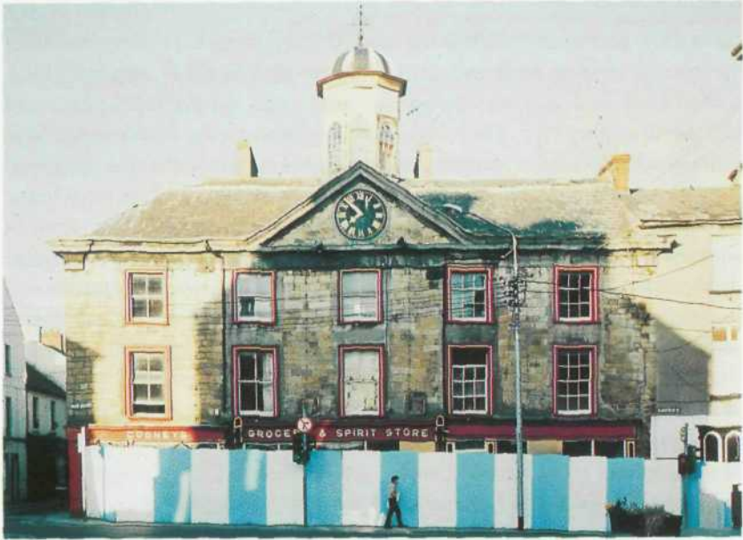
1. Main Guard, Clonmel. West elevation from O'Connell Street.
