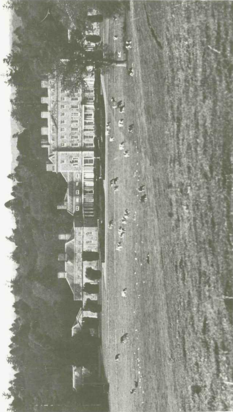
View of Carton from the Prospect Tower.
