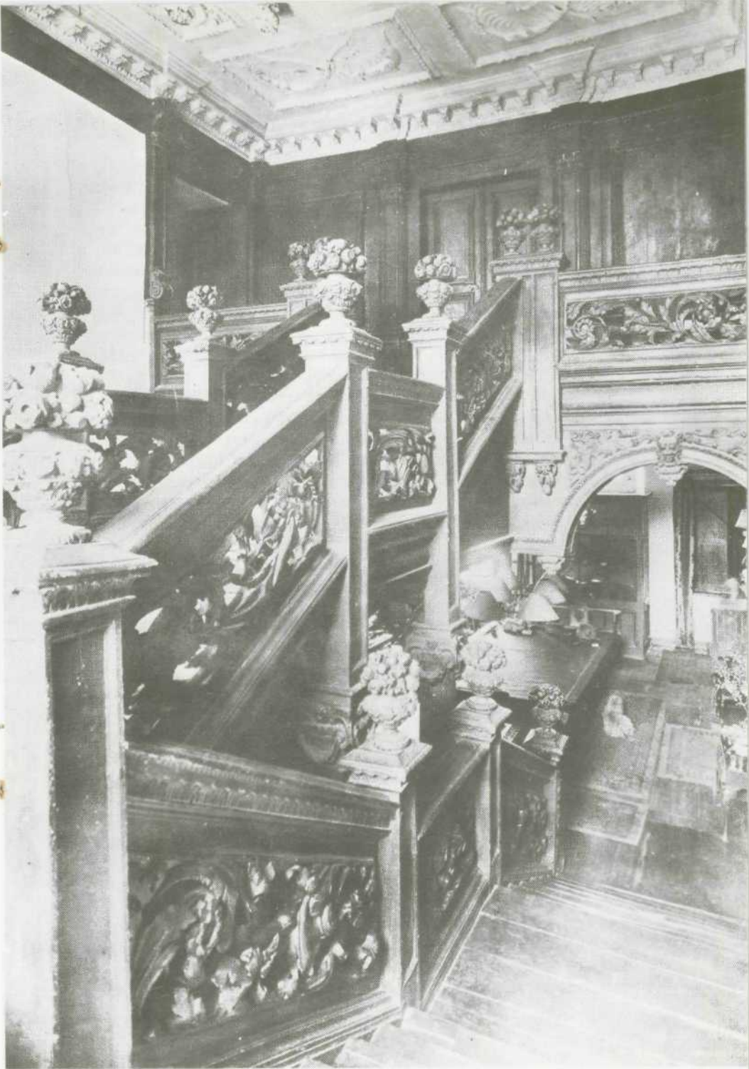
Plate 11: Staircase of Eyrecoiirt, Co. Galway, when still in situ (now stored in the Detroit Institute of Arts).
