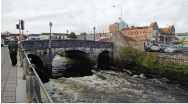
9 – South Gate Bridge
