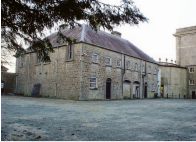
7 – East wing and courtyard prior to restoration, with light streaming through the ‘magic door’ in the colonnade, January 2007 (courtesy OPW)
