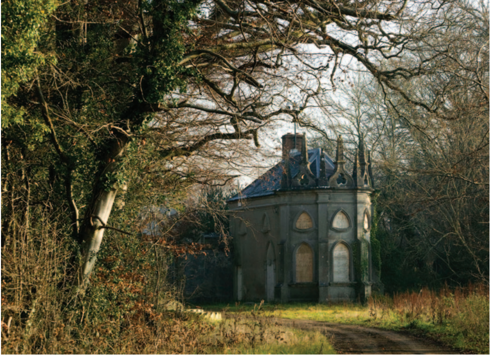
10, 11 – Batty Langley Lodge prior to conservation, December 2007 and after restoration, July 2016
