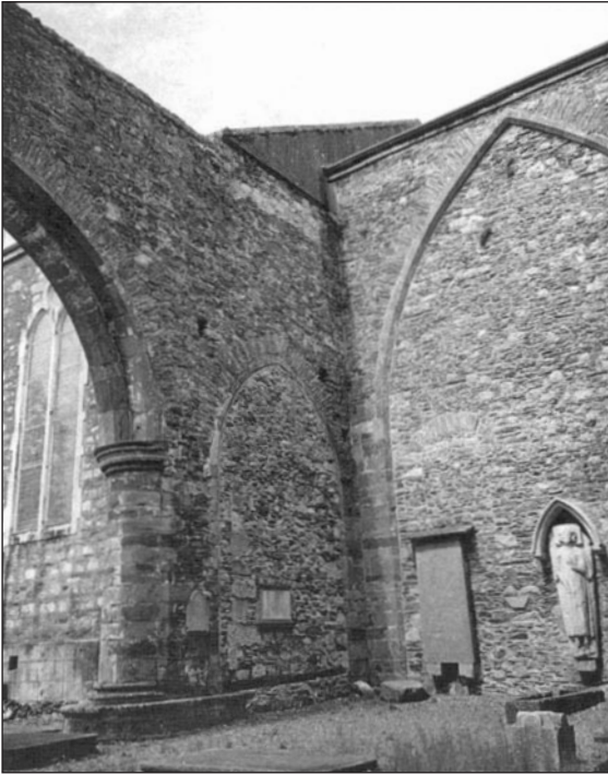
16 – St Mary's, New Ross: view from the south transept showing the blocked arches of the transept arch and the south aisle, with the later church on the left
