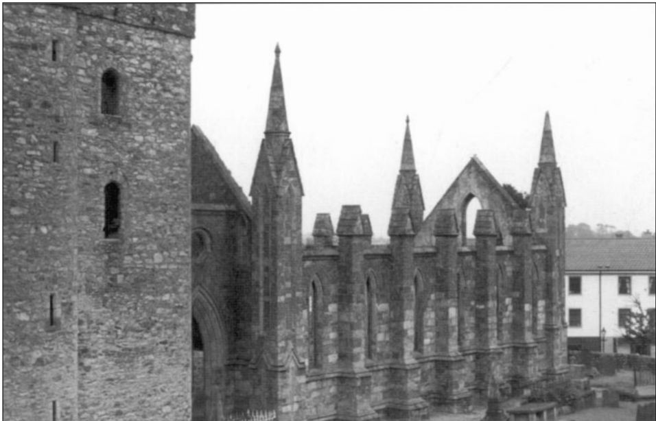
15 – St Selskar's, Wexford, showing the new church (attributed by the author to John Semple), built in 1826. The paler stone from the demolished chancel is reused in the walls.
