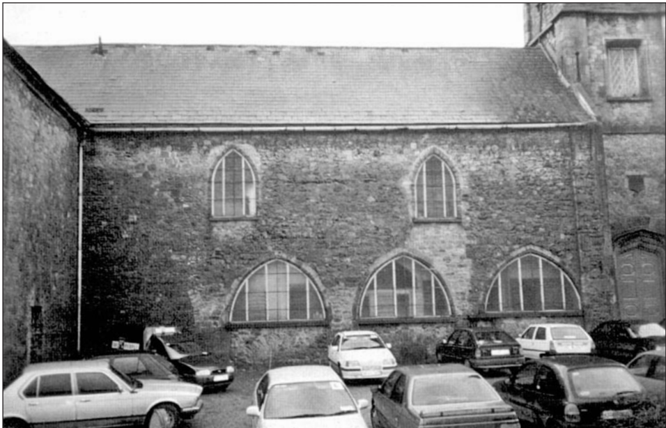
7 – St Mary’s parish church, Kilkenny: view from the north of the north wall of the nave showing windows inserted into the blocked aisle arcade
