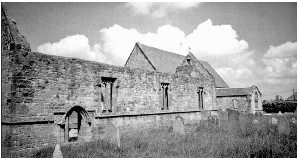
11 – St Mary's parish church, Callan, Co Kilkenny: view from the south-west showing the roofless south aisle with the re-roofed chancel behind
