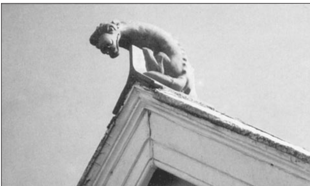
9 – Example of terracotta supplied from a catalogue: a ridge tile to a gable
