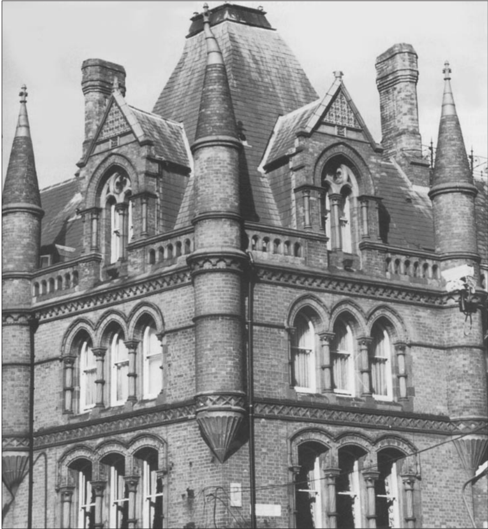
2 – South City Markets: detail of corner pavilion with pyramidal mansard roof and tourelles
