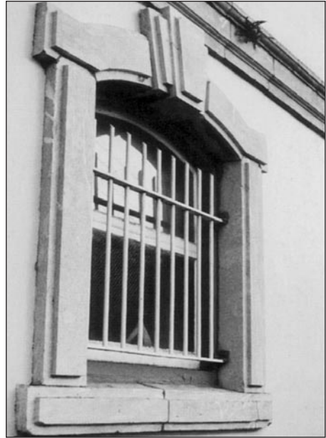
7 – Detail of river front, Custom House, Limerick, showing an upward break in the architrave of the second floor window (photo: Judith Hill)
