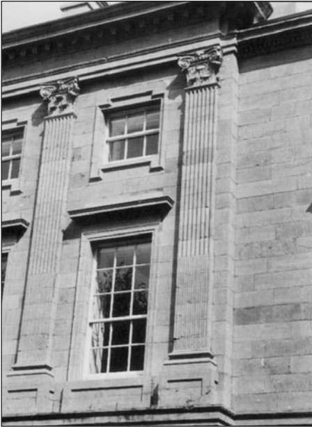
7 – Detail of river front, Custom House, Limerick, showing an upward break in the architrave of the second floor window (photo: Judith Hill)
