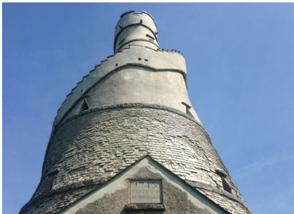
6 – Plaque over front entrance commemorating the builder John Glinn's work on the Wonderful Barn in 1743
