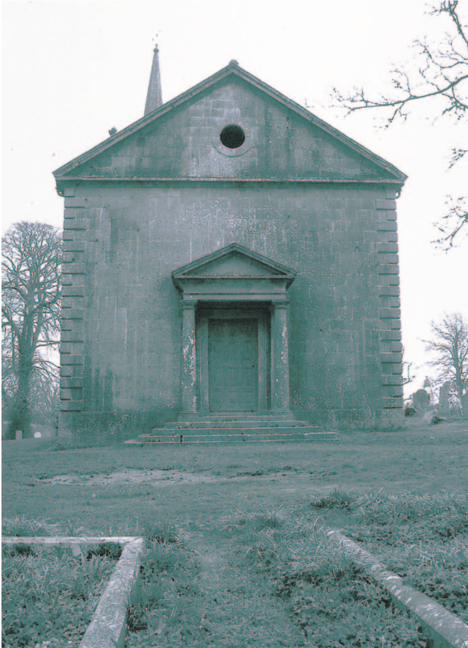
1 – Ardbraccan Church, county Meath The executed design is comparable to St Paul's Church, Covent Garden, by Inigo Jones
