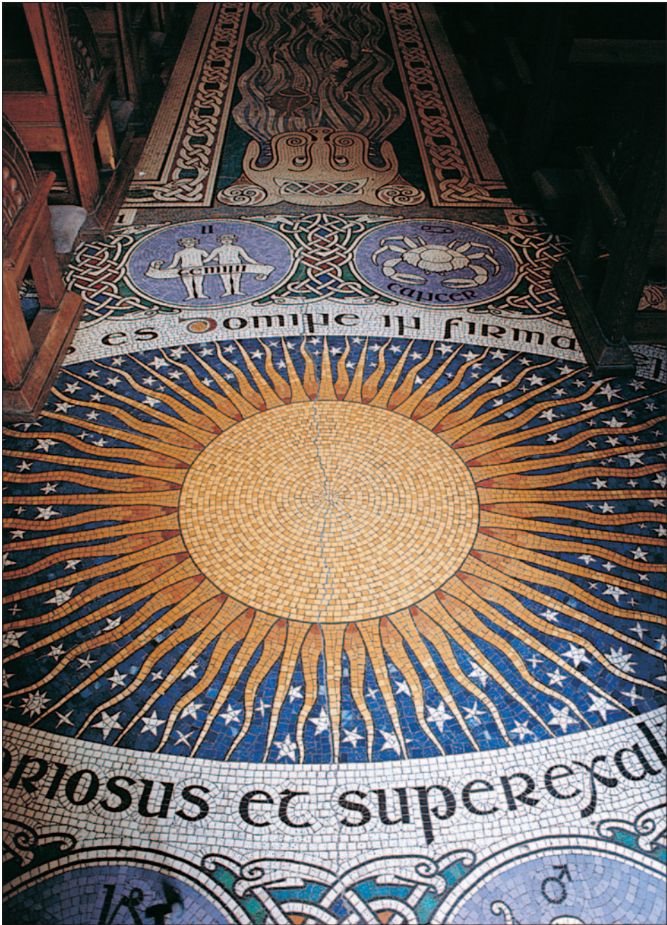
16 – Detail of nave floor by L. Oppenheimer Ltd
