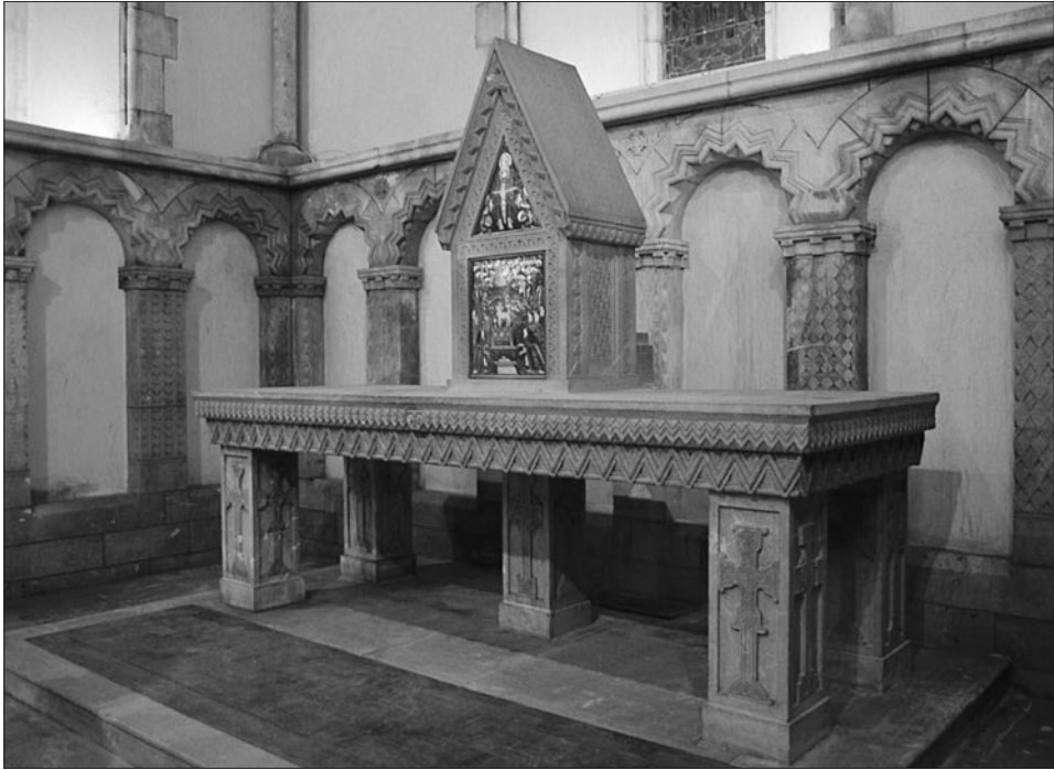
13 – View of the sanctuary with altar and east wall uncovered
