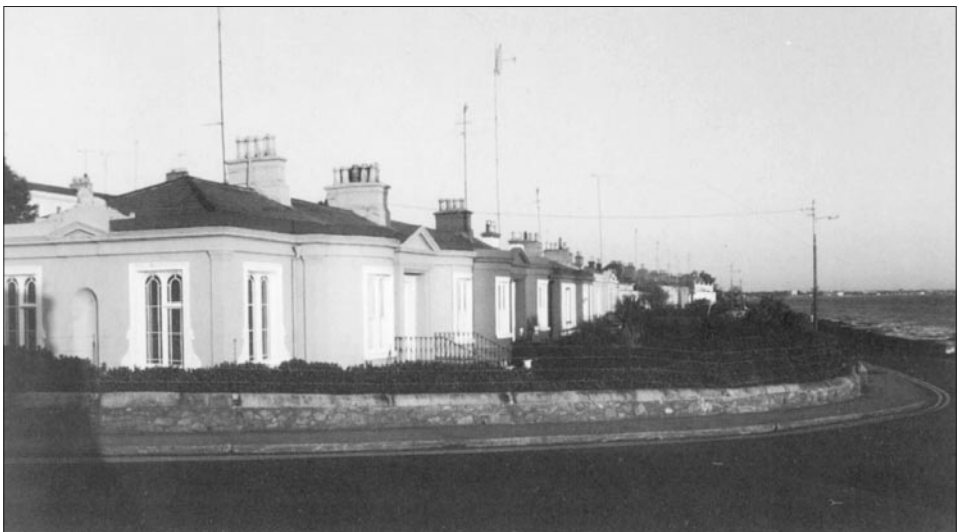
7 – Brighton Vale, Monkstown, Co Dublin view of the southern end showing some of the earlier houses (photo: John Stafford)
