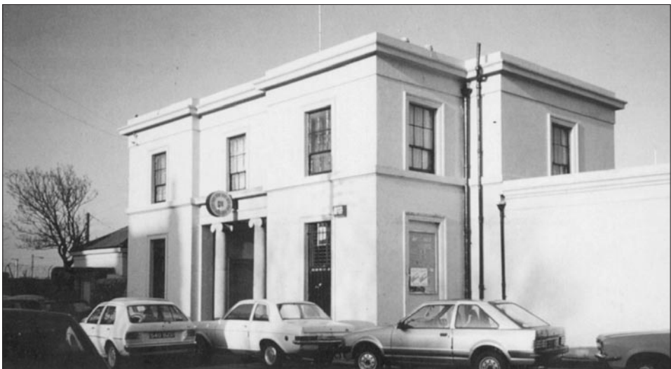
13 – Blackrock Railway Station, Co Dublin (1841) one of several buildings with a portico in antis feature
