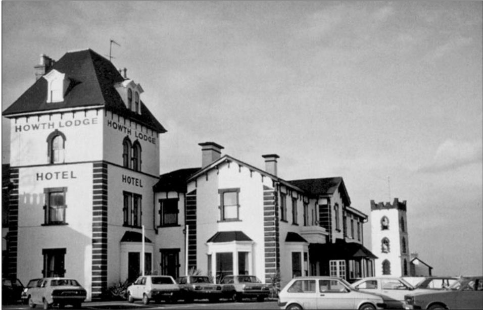
35 – Claremont (Howth Lodge Hotel), Howth, Co Dublin (c.1857), photographed c.1982 before the enlargement of the window openings; it was acquired for redevelopment in 1998
