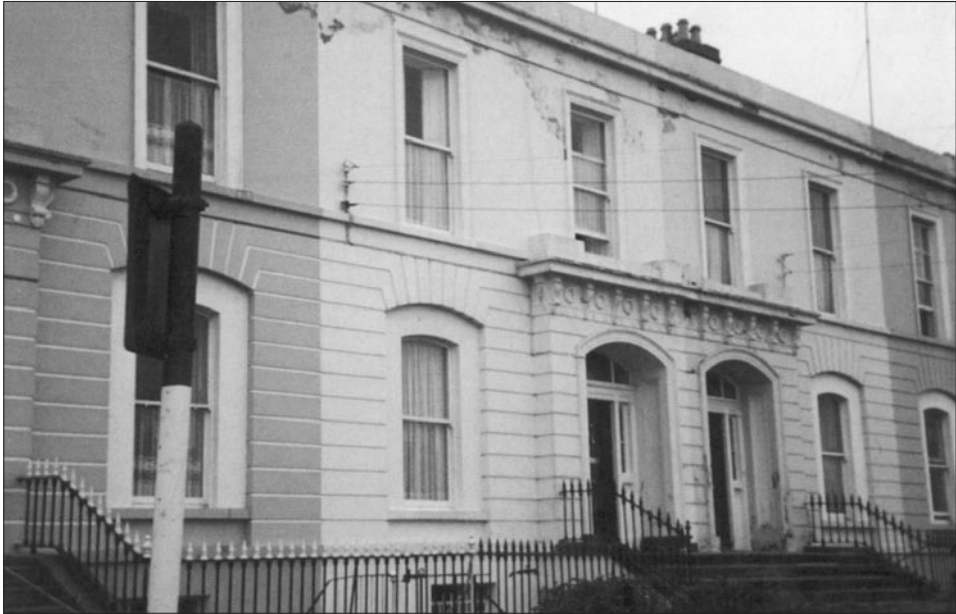
8 – Trafalgar Terrace, Monkstown, Co Dublin (1844-55) Mulvany lived on the terrace between 1864 and 1870
