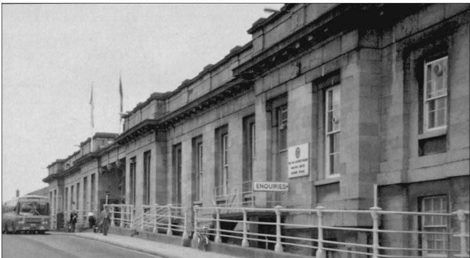
30 – Galway Railway Terminus photographed in 1982 before the removal of its sash windows
