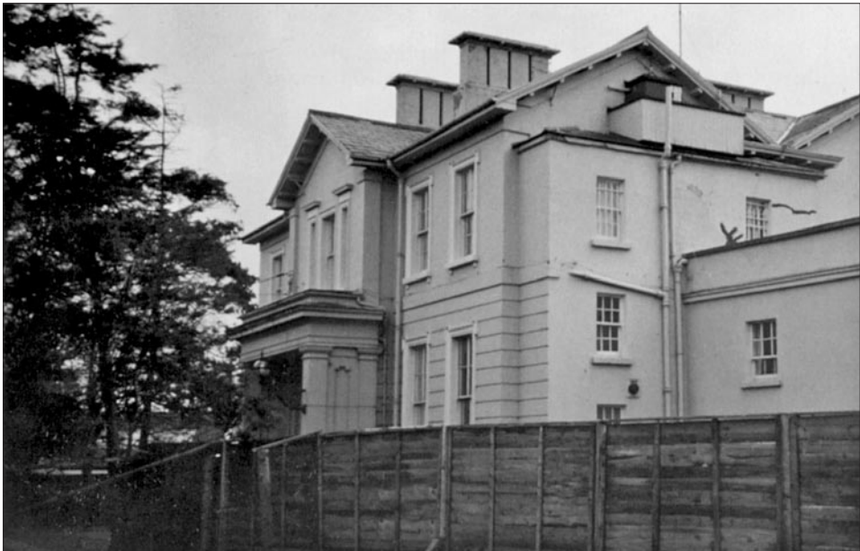
36 – Friarsland (now Glenard University Residence), Clonskeagh, Co Dublin, remodelled from an earlier house, Friarland, c.1859, with the rear elevation recast as a façade
