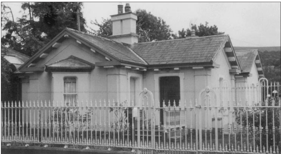
34 – Minella, originally Colville, Clonmel, Co Tipperary, gate lodge, probably the lodge for which Mulvany exhibited a drawing (by Raffles Brown) at the RHA in 1862 – a stucco version of the Mount Anville lodge
