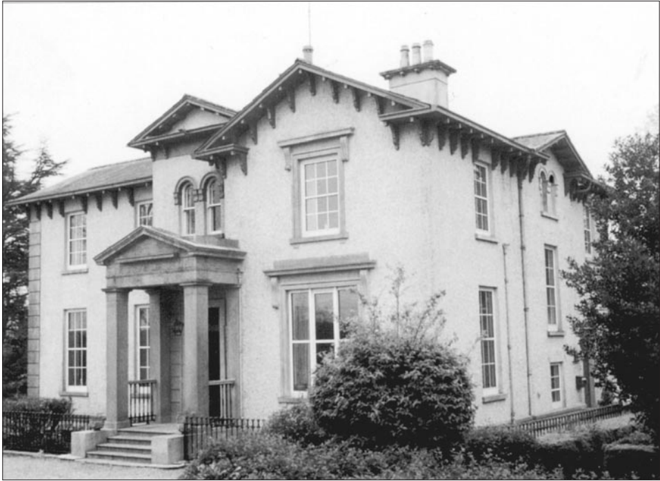
50 – Ballinagore, parish of Newtown, Co Westmeath (c.1850-54) an eclectic design combining some of Mulvany's 'free-style' motifs with classical elements
