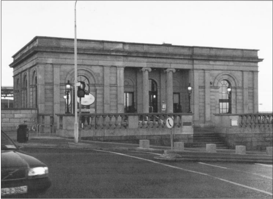
12 – Dun Laoghaire (formerly Kingstown) Railway Station, Co Dublin (1839-42) the channelled masonry of the lower wall surfaces is characteristic of Mulvany's work
